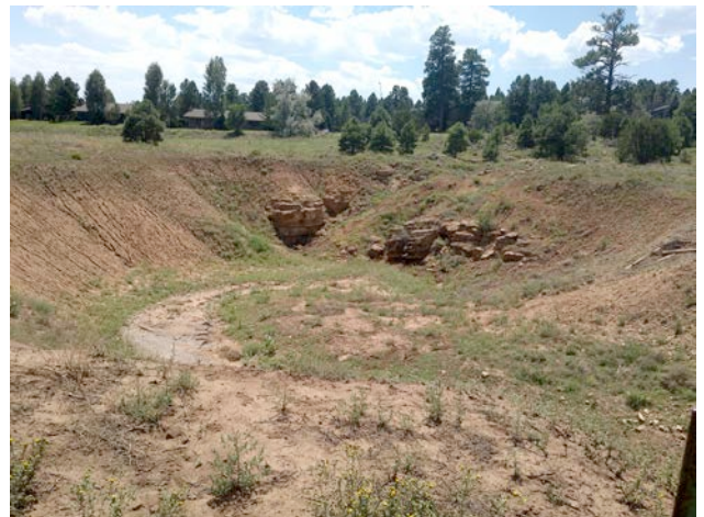
Figure 31. Photograph of Bottomless Pit, about 20 feet deep; looking south in August, 2018. Ledges at the south end of the pit are Kaibab Formation limestone. Fine, silty lake deposits and alluvium overlie the limestone. The limestone ledge is truncated on the left side (east side) by a fault that displaced the east side down (Fig. 29).
