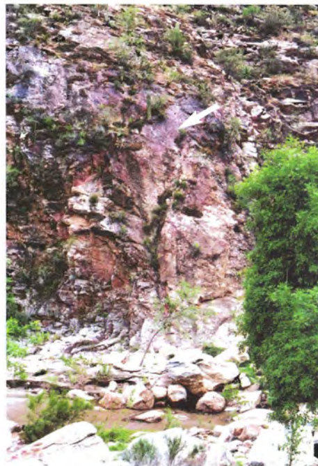
Figure SC 7.2. Closer view of the fault surface (arrow).
