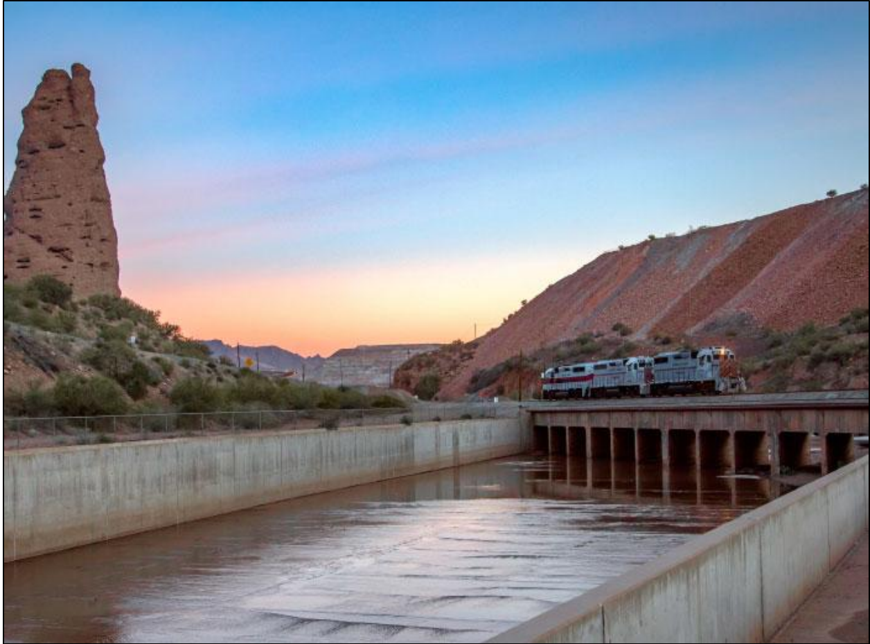
Figure 59. Concrete lining along Mineral Creek immediately downstream from the diversion tunnel outlet and Copper Basin Railway Bridge, looking north toward open pit ( photo from ASARCO website ).
