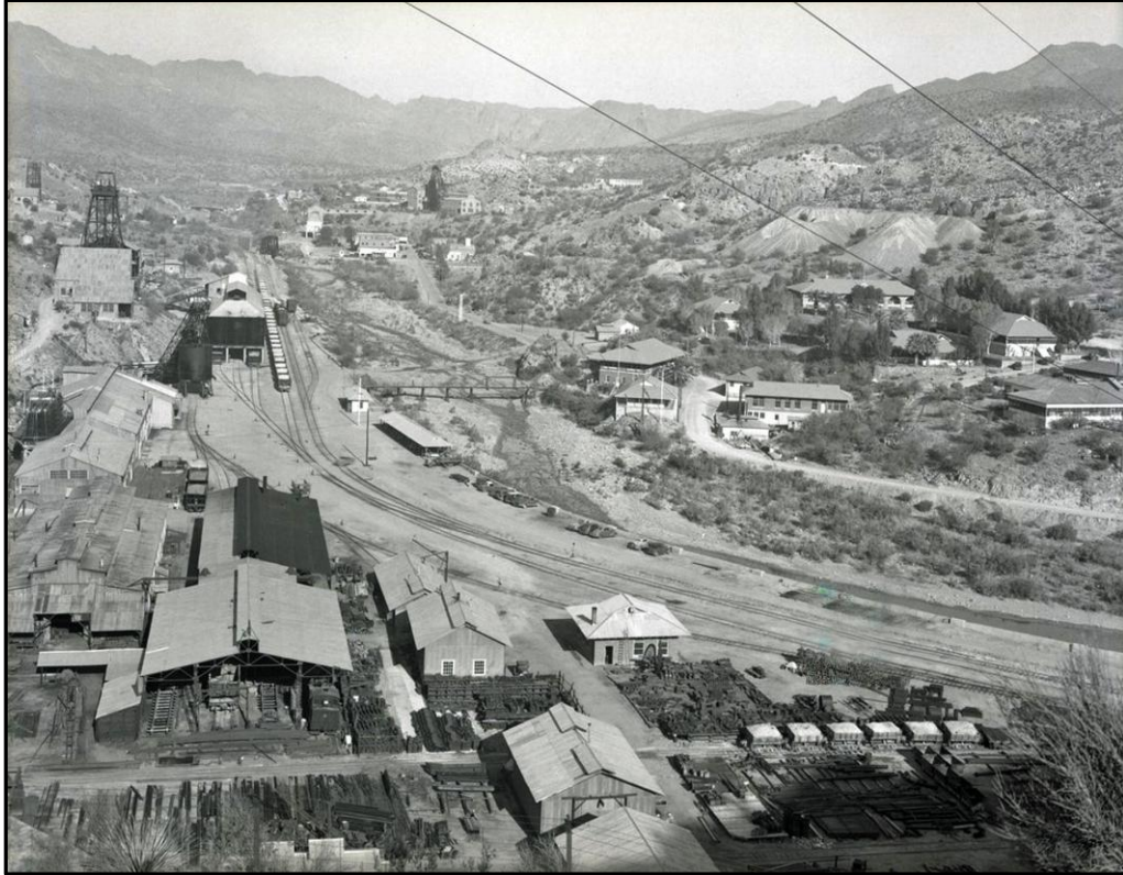
Figure 27. Headframe, crusher, ore bins, warehouses, and support facilities at the Ray No. 1 mine, looking north with town of Ray in the distance, circa 1930's (photo from Arizona State University Library Digital Repository).
