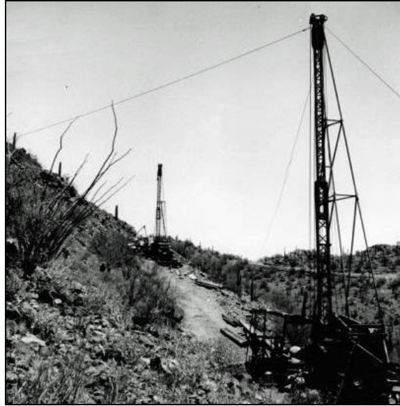
Figure 11. Churn drilling on Copper Girl Hill at Silver Bell (circa late 1940s). This form of early drilling employed a blunt-edge chisel bit attached to a string of drill pipe, which was raised by a cable or rope and allowed to drop, pulverizing the rock with successive blows (Photo provided by Arizona Geological Survey).
