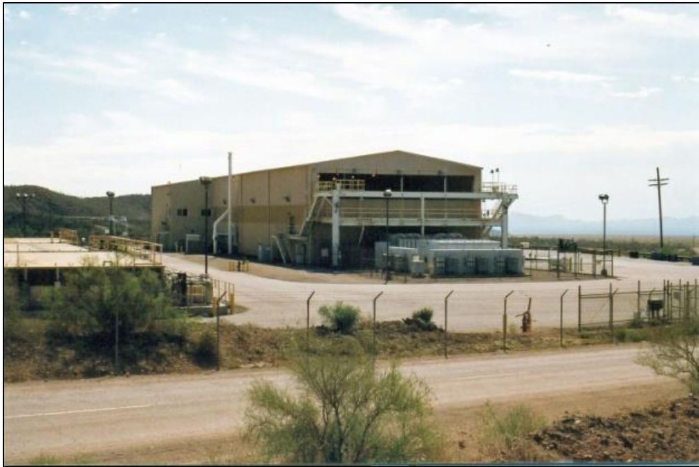
Figure 19. Electrowinning tank house at Silver Bell (Photo taken July 2004).
