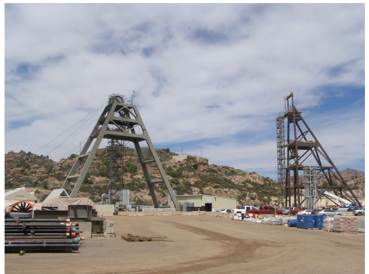
Figure 13. No. 10 (left) and No. 9 Shaft (right) at East Plant Site looking west (June 2015).
