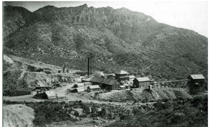
Figure 4. An overview of the Silver King Mine showing the loading chute, crusher, stacks of lumber and other buildings (circa 1880s) (2011-03-4268, ADMMR Photo Archive, Arizona Geological Survey).
