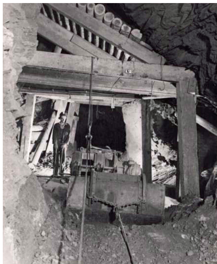
Figure 9. Miner operating a slusher at the Magma Mine (date unknown) (Photo provided by Magma Copper Company). Slushers are essentially a double-drum hoist attached to a scraper by a system of pulleys and cables that are employed to pull rock away from the mine face so it could be more easily loaded into ore cars.
