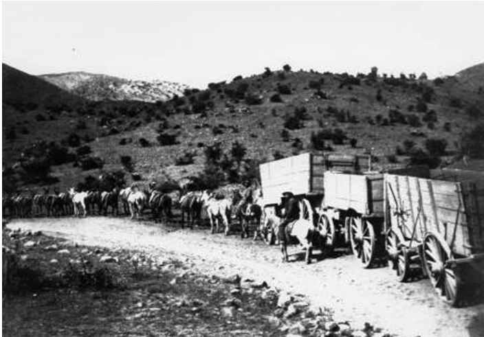
Figure 2. A wagon train of three ore carts pulled by many mules hauls ore from the Silver King Mine to the Pinal City mill (circa 1880s) (2011-03-4270, ADMMR Photo Archive, Arizona Geological Survey).
