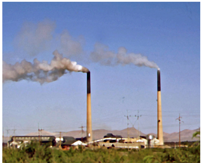
Douglas Smelter (Environmental Protection Agency, June 1972).
