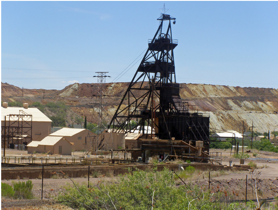
The Campbell Shaft located about 0.5 miles southeast of the Lavender Pit
